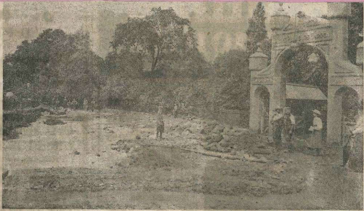
View in Bridge Lane
